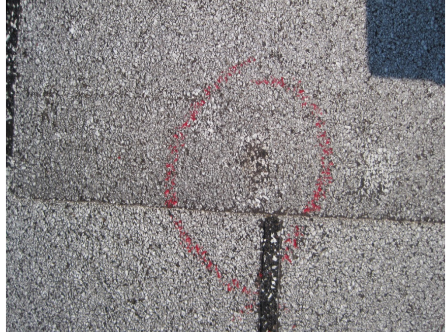
Close up of hail damage in test square
